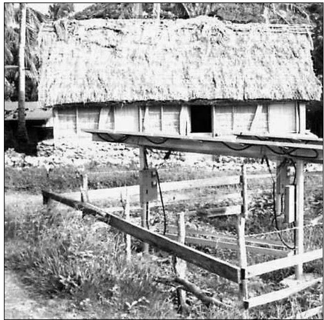
Solar battery charging station for fish refrigeration and other community needs (Batanes, Philippines).
