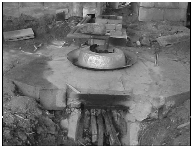
Training enabled Ban Mae Pa Haen community members to build an energy saving stove to generate curing steam for community services (Sunsai District, Chiangmai Province, Thailand).
