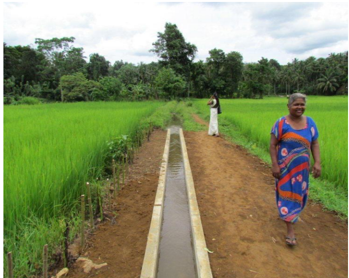
Cultivated paddies flourish with upgraded water channels that bring water during extended dry seasons as well as help to reduce flooding. Photo: Tharuka Dissanaike, 2012
