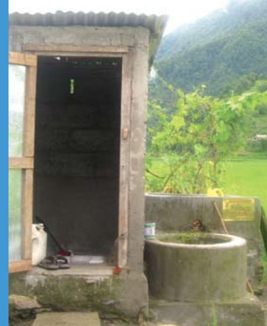
Toilet - attached water hyacinth-fed biogas plant
