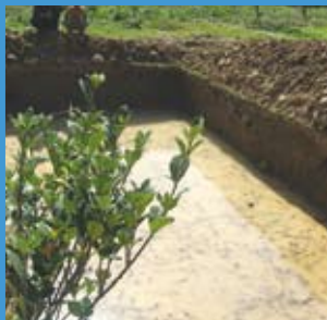
Digging earth for biogas dome
