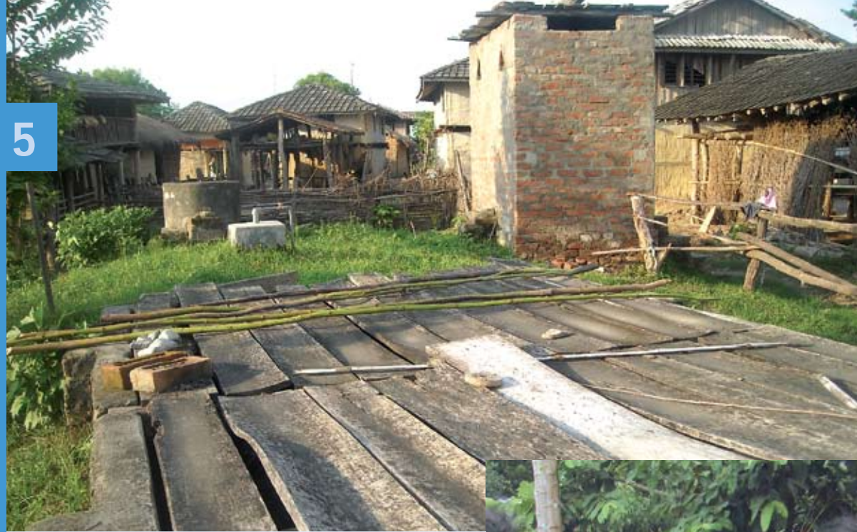
Inlet, gas outlet and slurry outlet of a community biogas plant in Sarlahi
