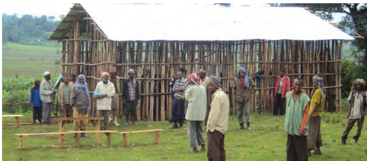
Building under construction to be used for fattening livestock, COMDEKS Ethiopia
