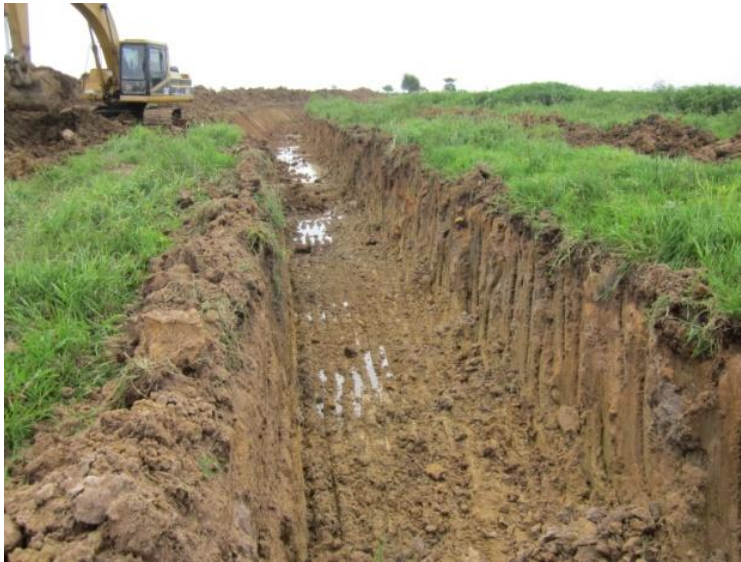
Figure 2 Canal rehabilitation works for improved irrigation and drainage in the target areas. 2012. Photo: Courtesy of SGP
