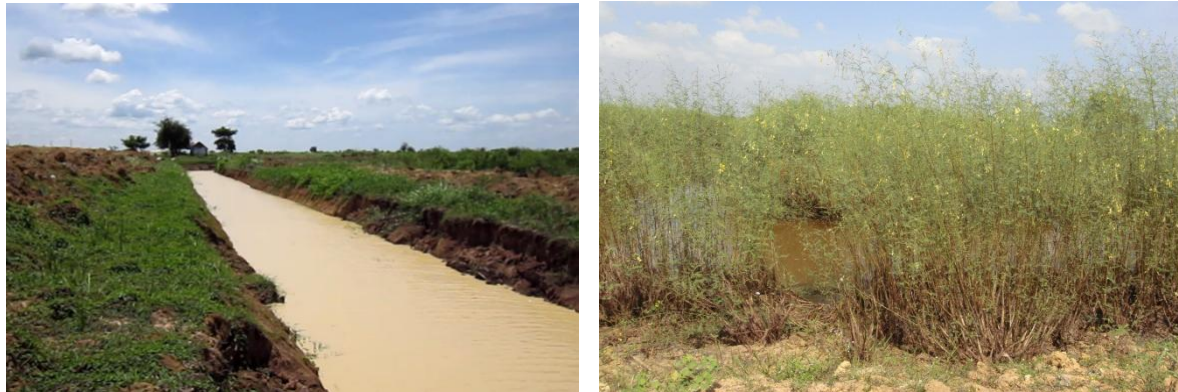
Figure 3 and 4: The rehabilitated conservation lake and fish refuge (left) with stabilising planting along the embankments 1 year after restoration (right). 2013. Photo: Courtesy of SGP Cambodia.
