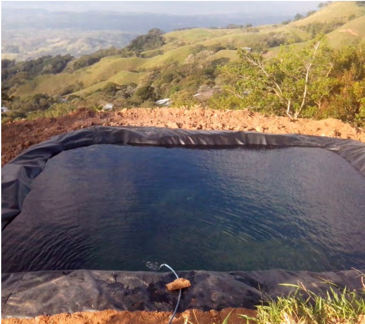
A reservoir in the mid-river basin provides water for irrigation, animals, and other uses, COMDEKS Costa Rica
