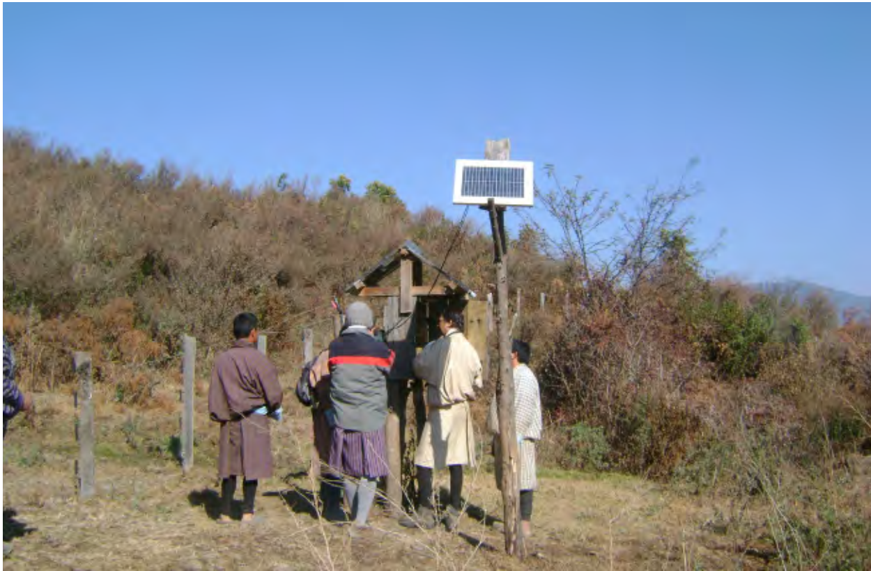
Installing solar fencing to mitigate human-wildlife conflicts, Yenangbrangsa, COMDEKS Bhutan
