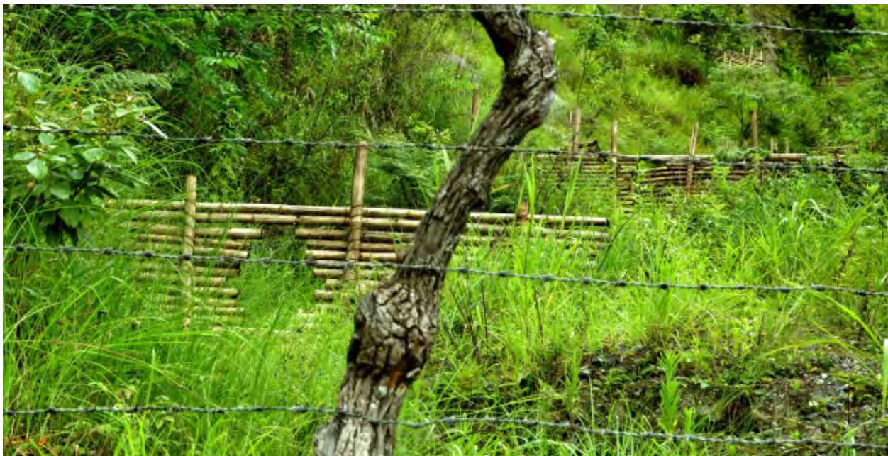
Bamboo check dams for erosion control at Pemochojay Ropta, COMDEKS Bhutan
