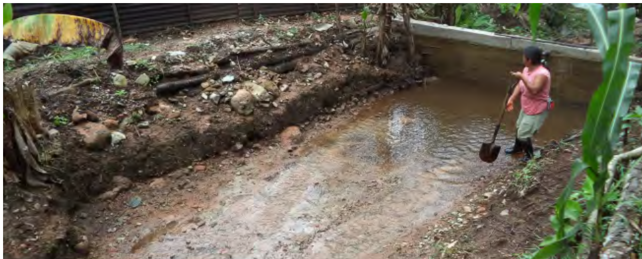
Construction of an aquaculture pond, Santa Rita, COMDEKS Ecuador
