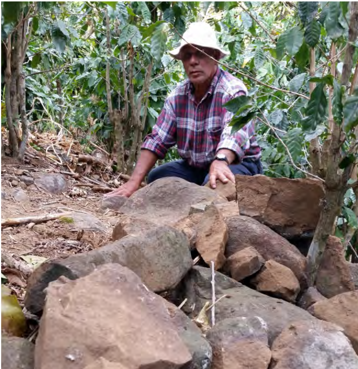
Inspecting a stone wall used to prevent soil erosion on slopes, COMDEKS Costa Rica
