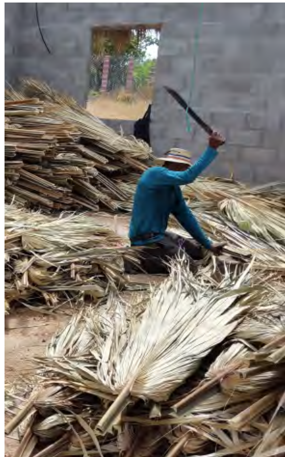
Preparation of palm leaves for roofing, COMDEKS El Salvador
