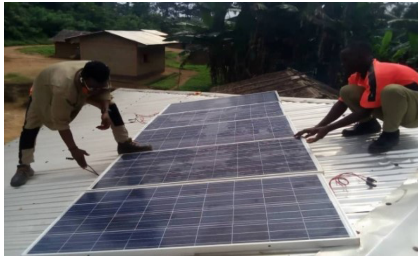
Technicians installing solar panels
