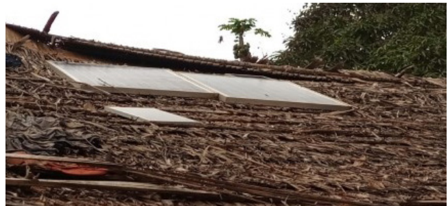
Solar panels installed on the roof of a home
