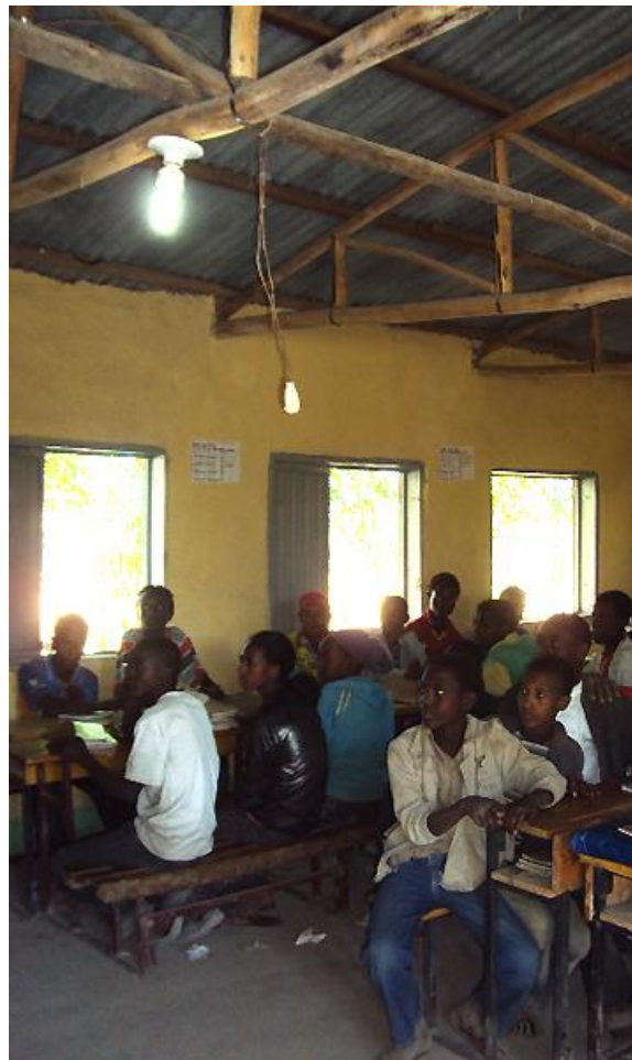
Solar electric light in school, Oromia
