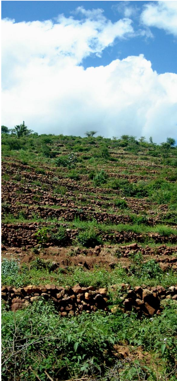
Stone bund constructed to prevent land degradation, Dire Dawa
