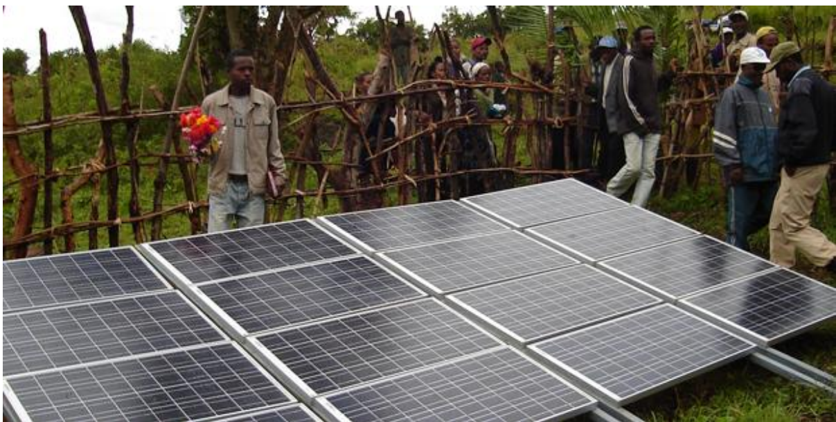
Solar panel installation, SNNPRS
