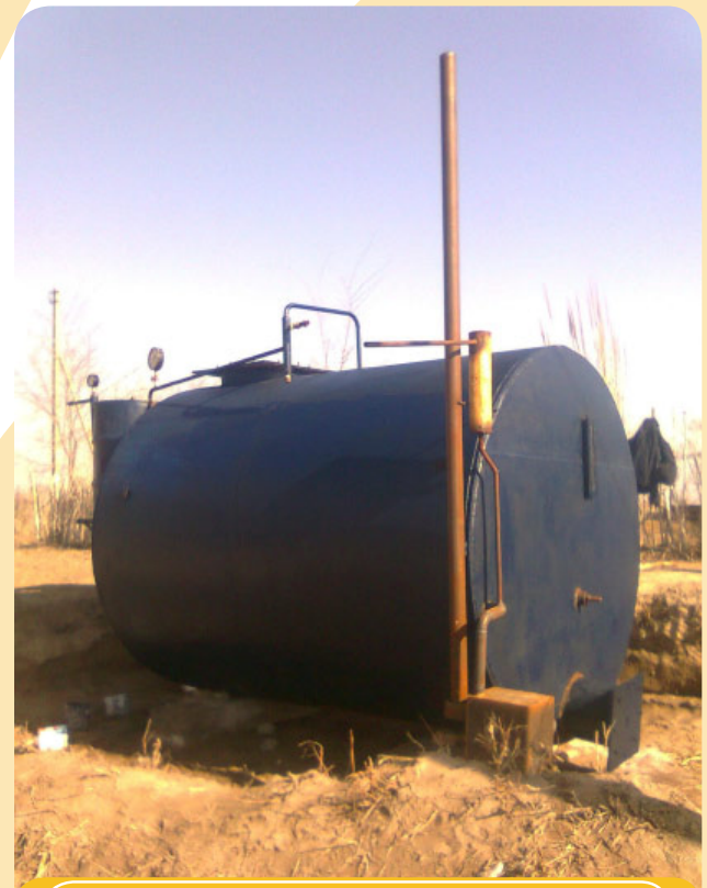
Biogas construction works (Photo by Atabek Atamuratov)
