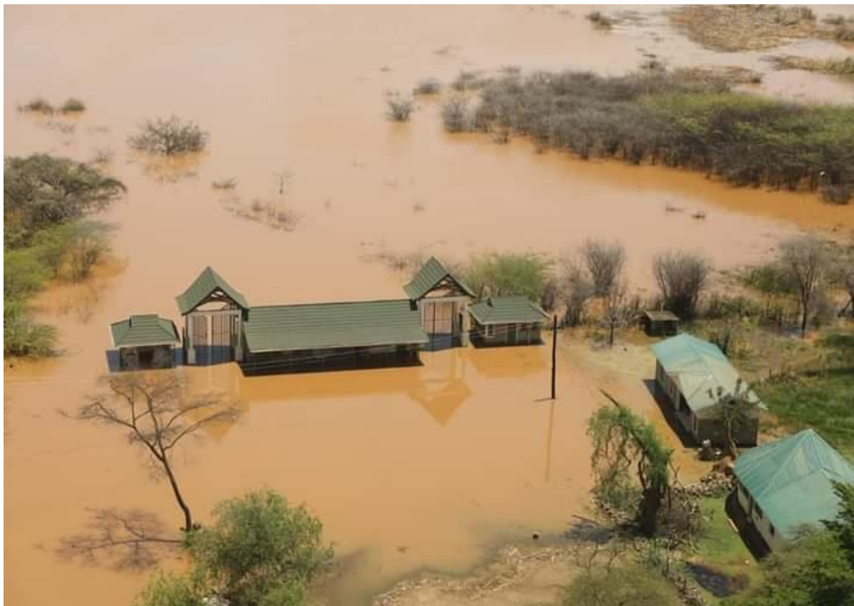
Aerial view of a submerged administration block at Lake Bogoria©James Kimaru
