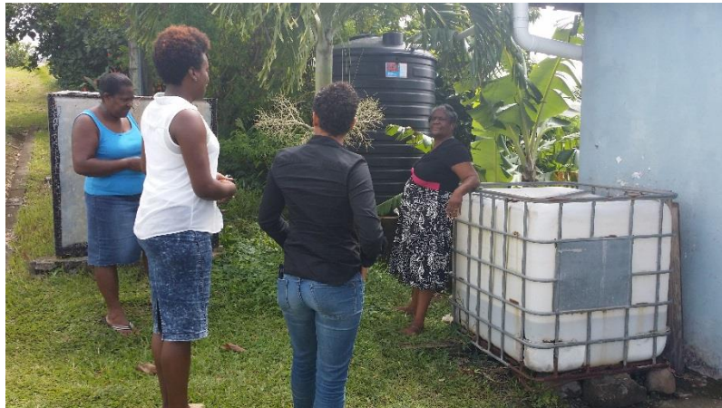
Rain Water Harvesting System (Bouton, Soufriere)
